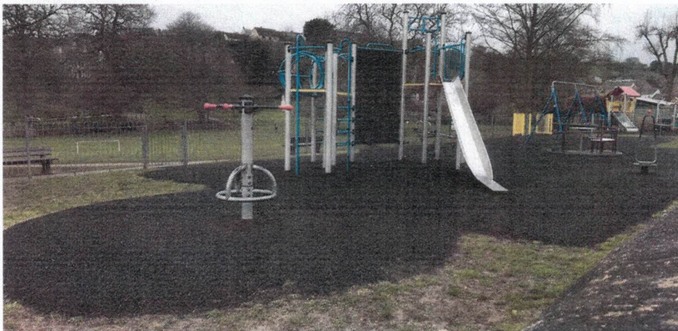
Example of correct installation. (Crediton)
